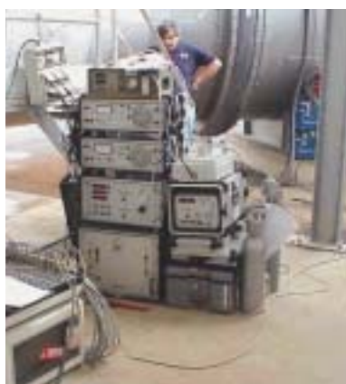
Equipment used by APAVE to test the post-combustion unit.
